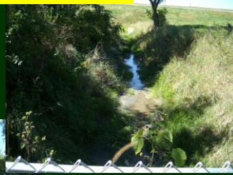
Ditch entering property from the West
